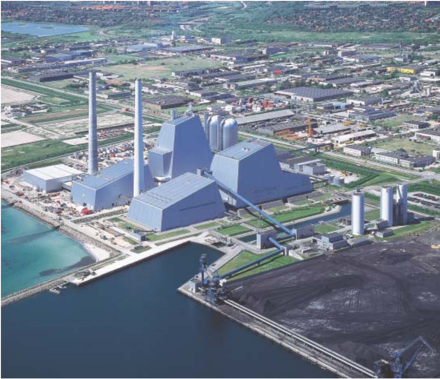
Avedøre 1+2 plant and the two accumulator tanks (in the middle behind the plant)
