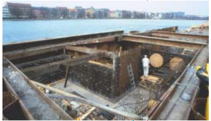
The pipe network going down deep ...
