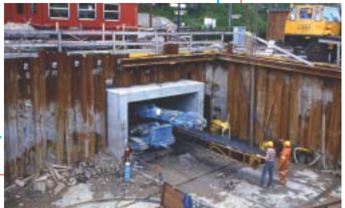
... under the railway system
